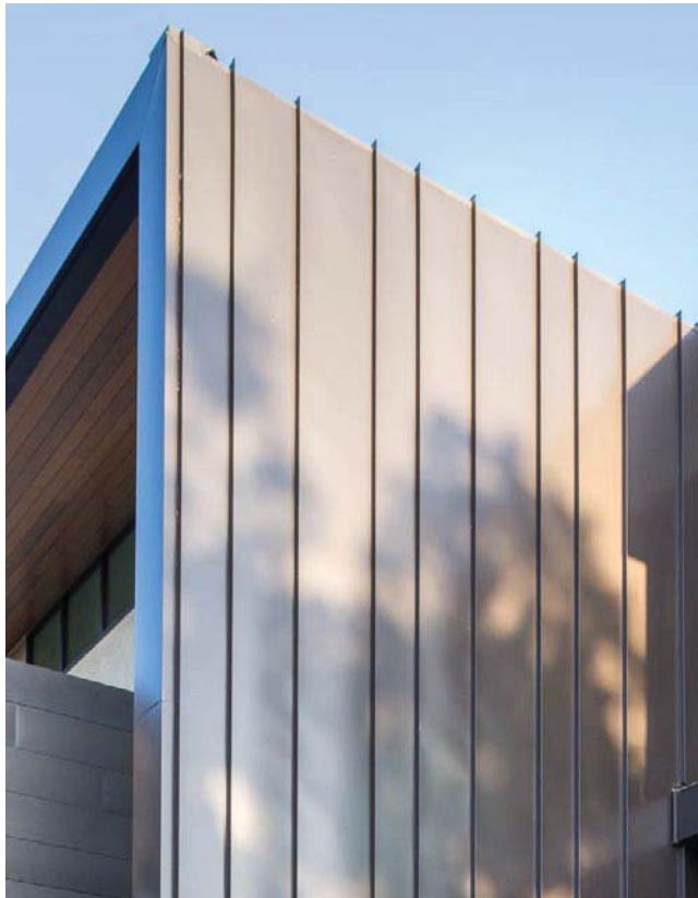
STANDING SEAM METAL CLADDING
